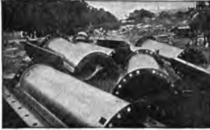
Fig. 311—Showing Steel Semi-Cylinders for the Marconi Tubular Mast.
